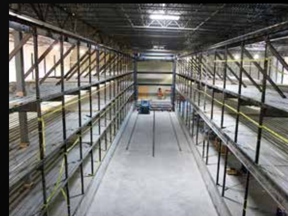
Robotic Parking System – High-Speed Vertical Lifts 7-level, high-speed vertical parking garage stores 325 cars. Programmable controls ensure uninterrupted operation. Lifts send and retrieve automobiles at a rate of 400 FPM.
